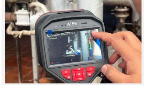
Gas Leakage Detection
